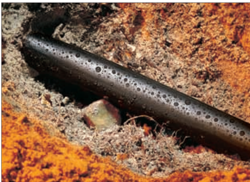
TREDUX HA47 – application below ground.
