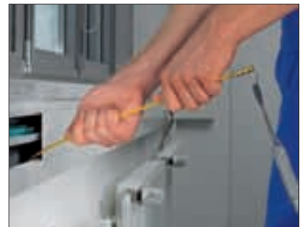
Installing cables through trunking. No problem with Cable Rod.
